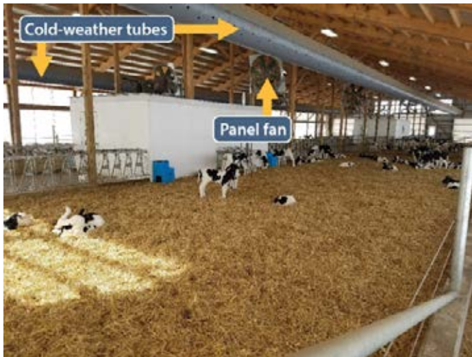
Figure 1: This calf barn uses natural ventilation in conjunction with cold-weather positive pressure tubes and panel fans. This system works only in curtain sidewall barns because the panel fans rely on open curtains to draw in fresh outside air during warm weather.
