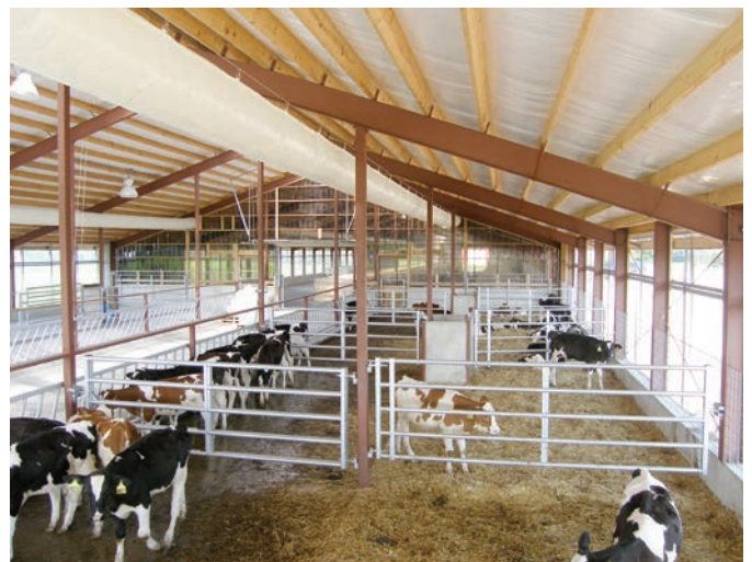
Picture 2: Notice the 18 inch height of the knee wall. Lower walls create better air flow at the level of the calves. Curtains are split 2/3 on bottom and 1/3 on top. They roll from the top down and bottom up, meeting in the middle.
