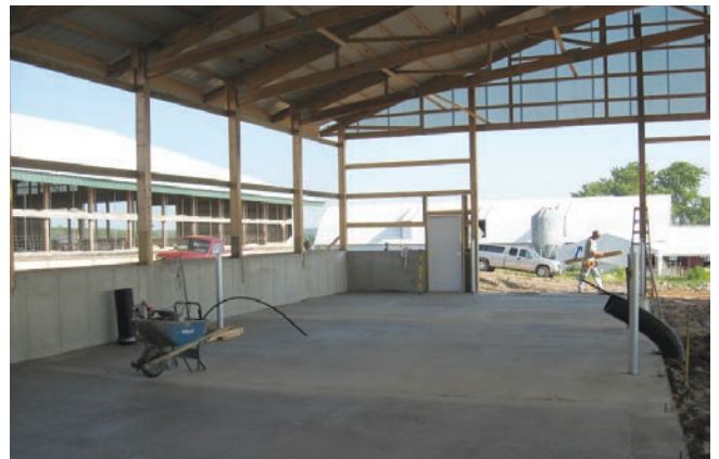
Picture 1: 4 foot tall concrete walls reduce ventilation at the level of the calf.
