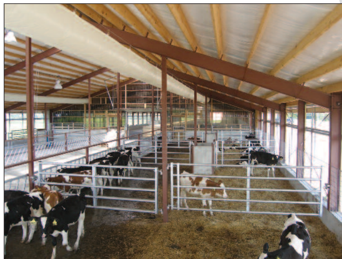
Positive pressure tube ventilation system in group housed calves.
