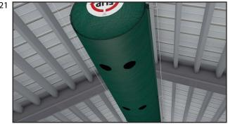
In this position, air flows only through the series of large-diameter holes at the bottom,
