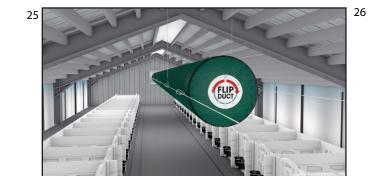
The simple steps for rotating FLIP DUCT® are performed only twice per year, once in spring – in anticipation of warm weather, and once in fall – in anticipation of cold weather.
