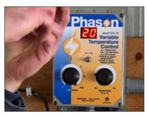
**Remove face plate**First, loosen the 4 corner screws and remove the face plate.
