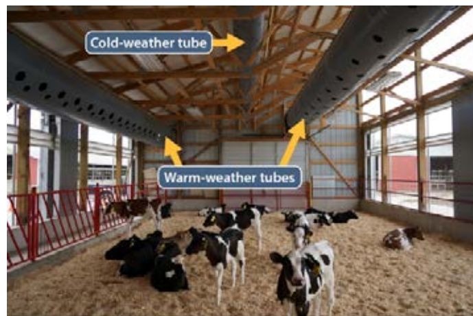
Figure 2: This calf barn uses natural ventilation with a central cold-weather tube and two warm-weather tubes. This system works well in solid sidewall barns because the tube fans deliver fresh outside air.
