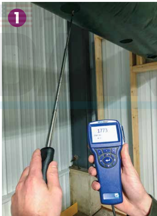
A hot wire-style air speed meter is used to measure air speed and volume from a positive-pressure tube.
