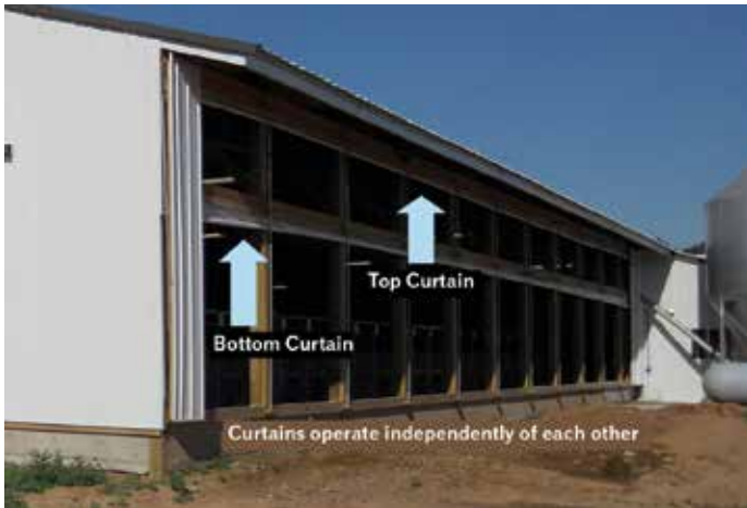
Picture 1: Splitting the curtains so the top and bottom halves move independently of each other creates flexibility for varying weather conditions.
