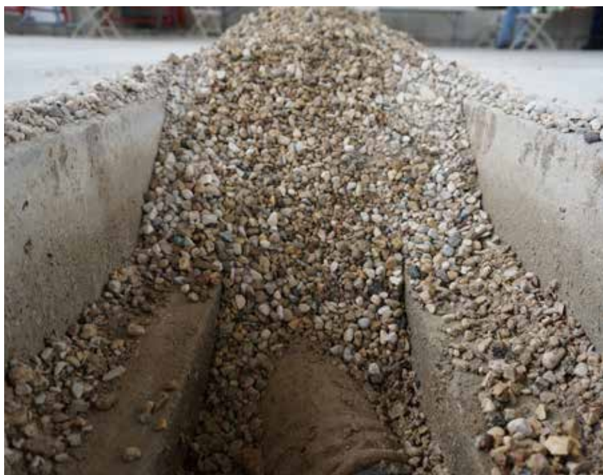
Picture 3b: Aggressive concrete slopes rapidly move liquid waste to a centrally located drain tile.
