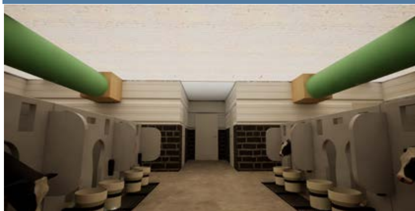
AN INTAKE BOX IS BUILT UP THROUGH A HAYMOW IN ORDER TO BRING AIR INTO THE BARN
